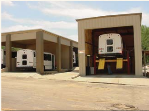
New bus inspection and water testing bays
